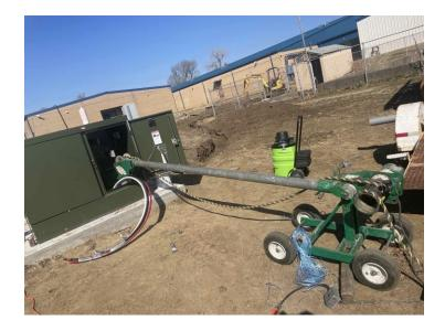
Pulling new power lines to new transformer set by PSO
