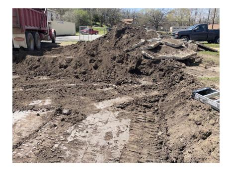
Existing concrete and soils were removed to a depth of 2ft below finished grade.
