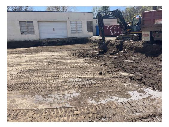
Soils removed to subgrade, ready for import of new select fill
